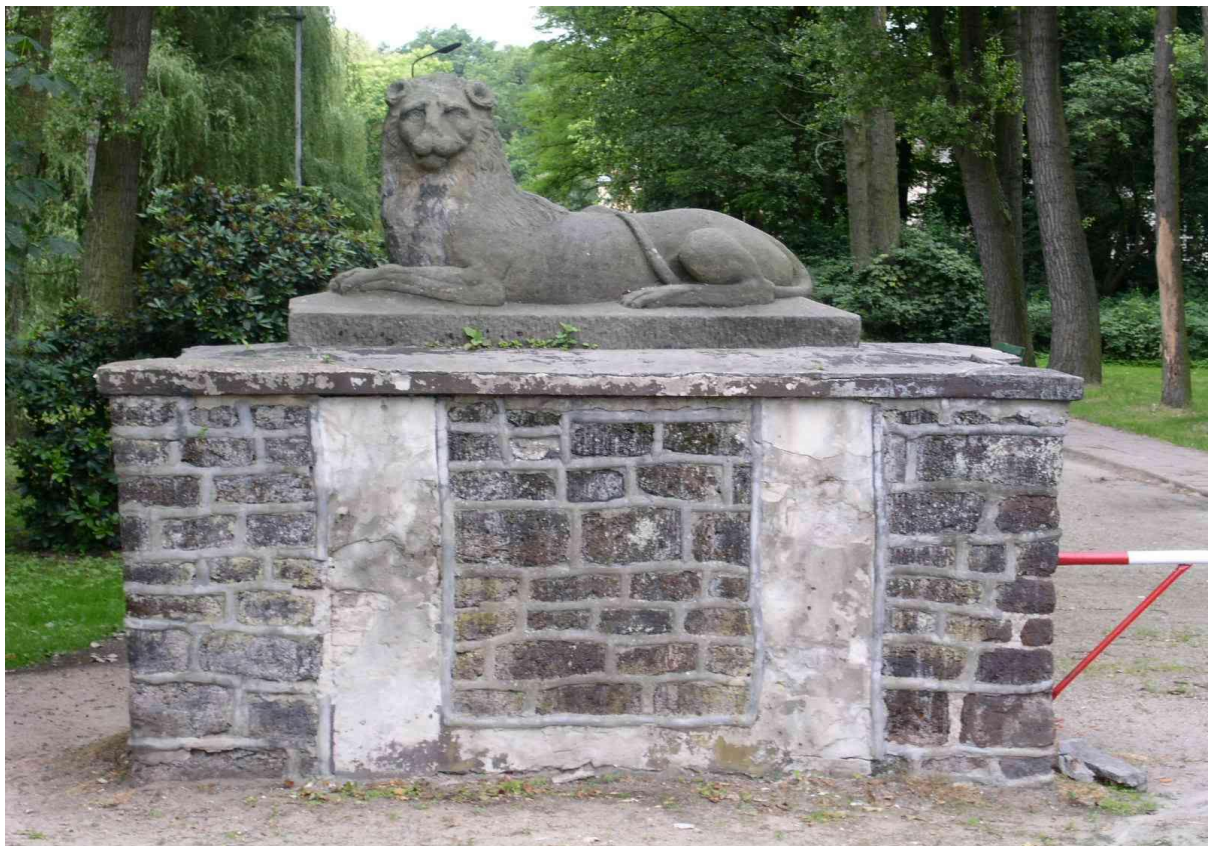
Fig. #F1 (B4 in [10]): The wall constructed from the "paddock ore". The above is all what remained until today from the former medieval fortification walls of the town Milicz. (Only that these walls in past stood in different locations than the
