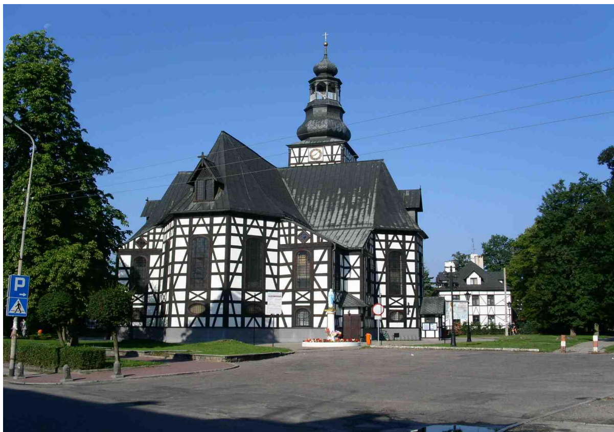
Fig. #G2 (B1 in [10]): The church of St. Andrea Bobola (i.e. "Św. Andrzeja Boboli") in Milicz - former Evangelical church. This church was constructed in the architectural style which in English is called the "tudor" style (in Poland it is usually known under the name of "mur pruski" what translates as the "Prussian
